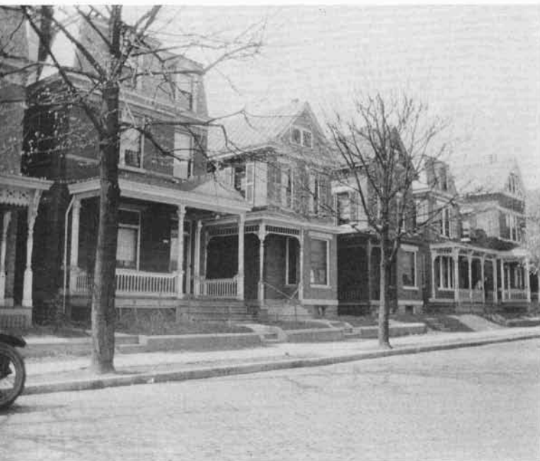
Narrow row houses built in the early twentieth century, such as these on Williamson Place, can be found on many of the streets in Section 28.
